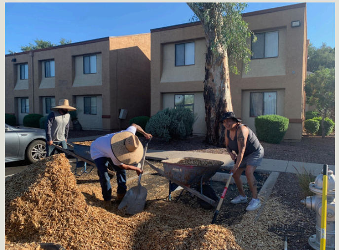
CST member Virginia Mireles and the Barrio Restoration crew at work
